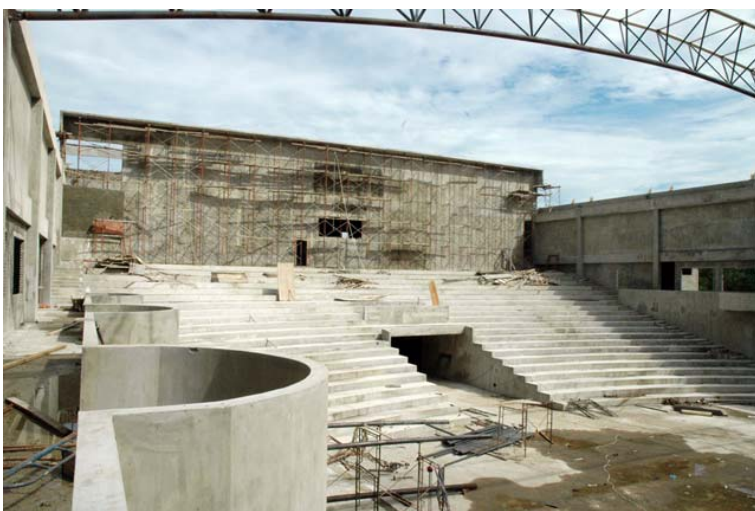
Picture above shows the auditorium under construction.
